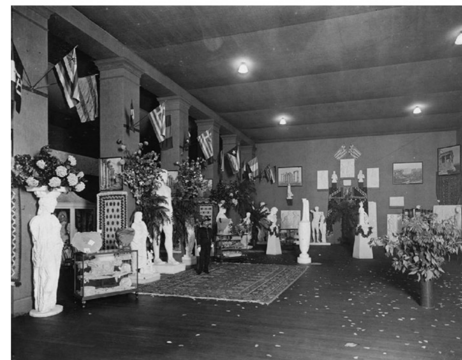
Interior of the Greek Pavilion
